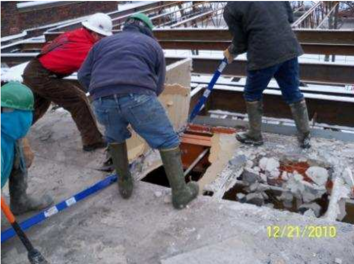
Annex roof removal work begins
