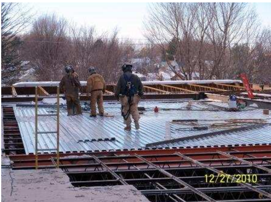
Continuation of roof removal and new decking installation
