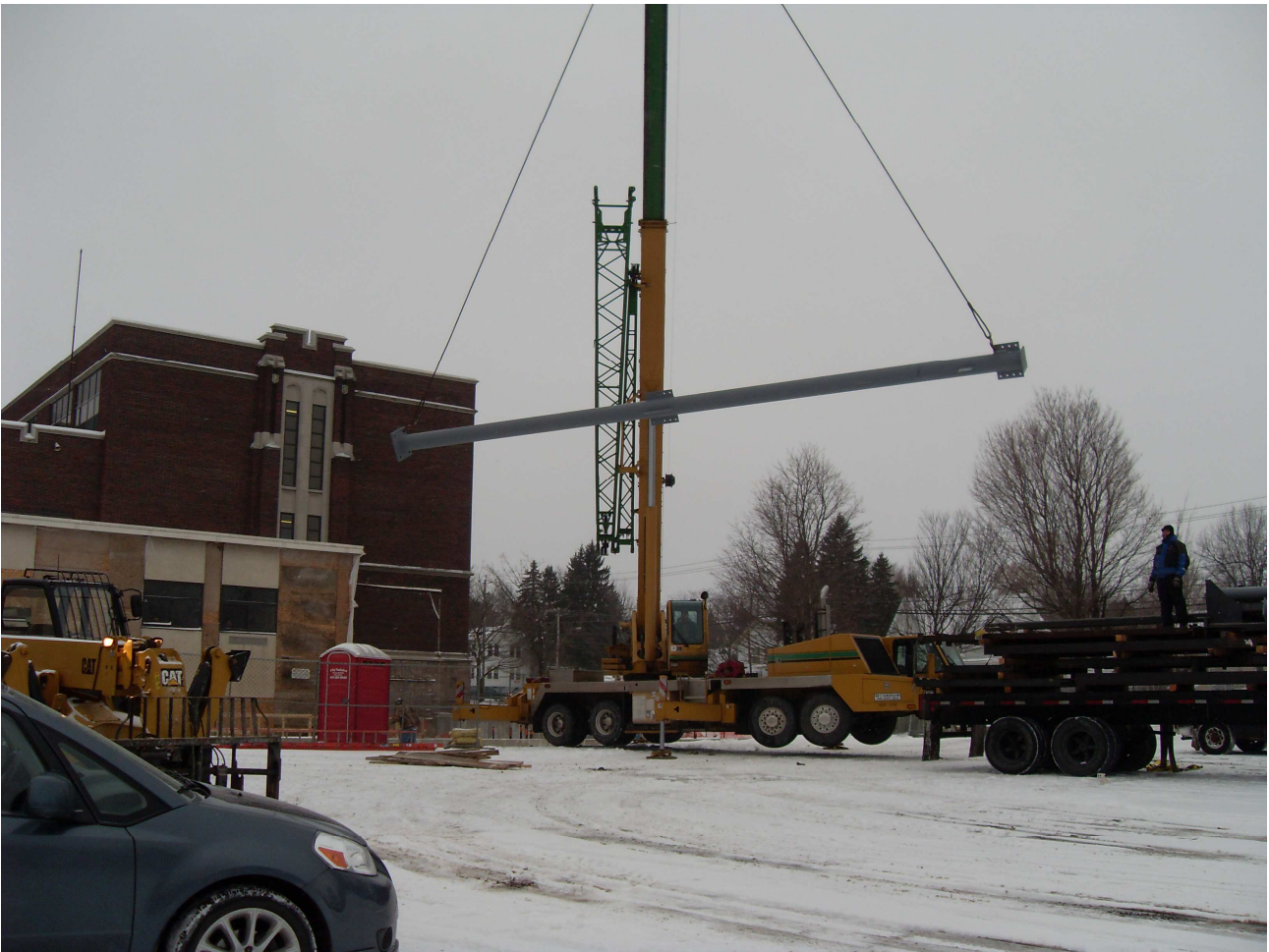
Structural steel at the Middle School is delivered and installation begins
