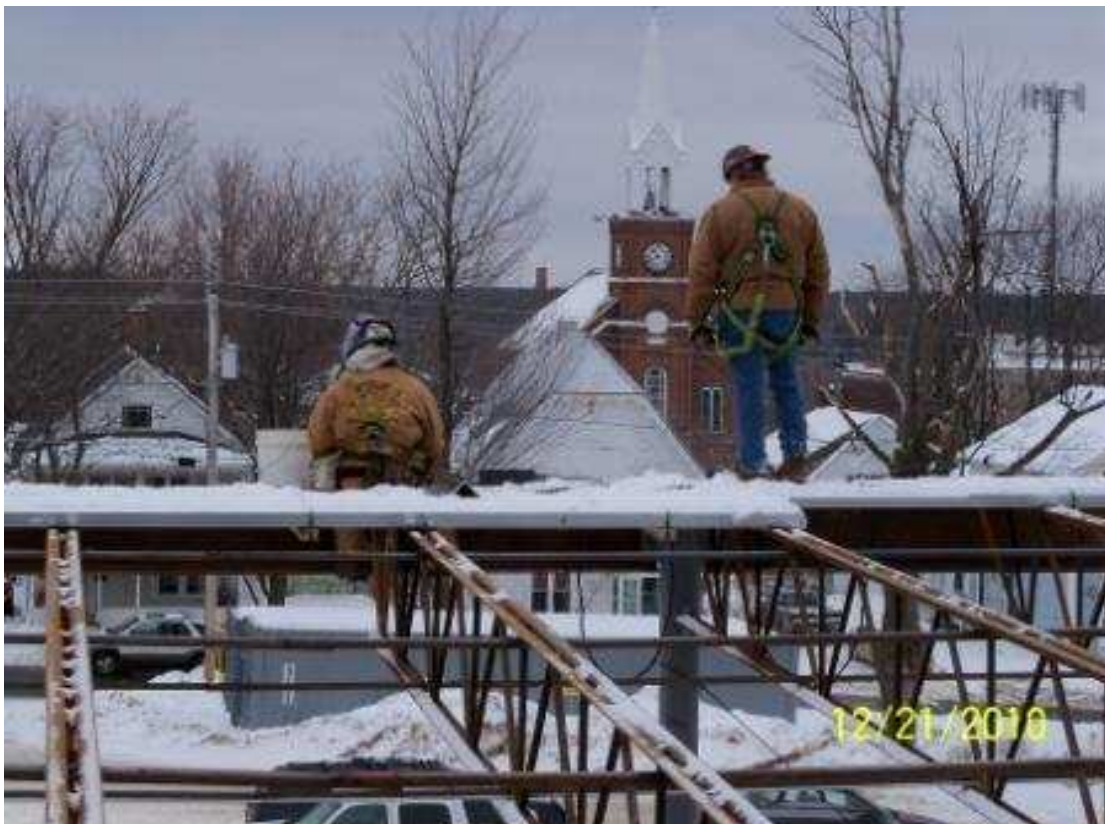
Middle School structural steel and connection work
